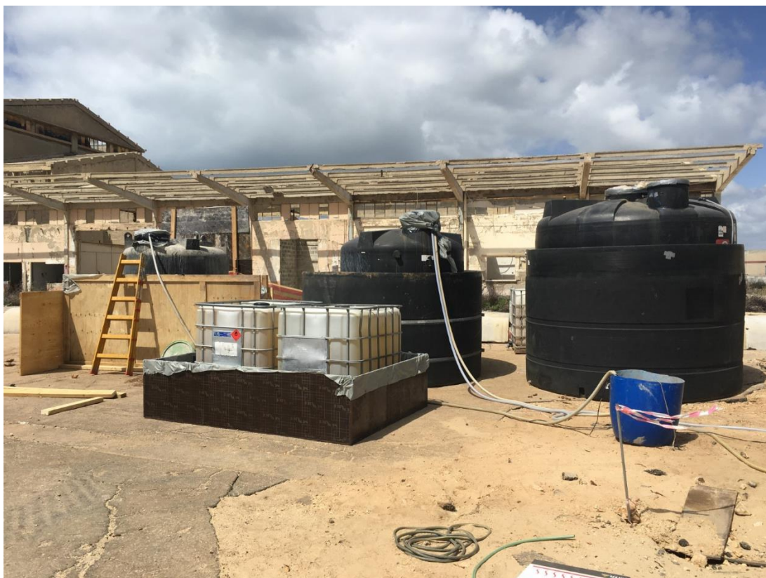
Figure 38. Condensate tanks in front of the pile
