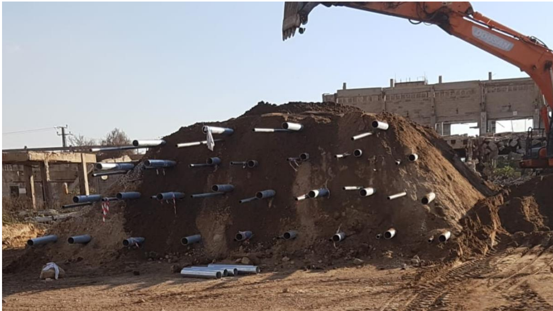
Figure 26. Building phase of the thermal pile
