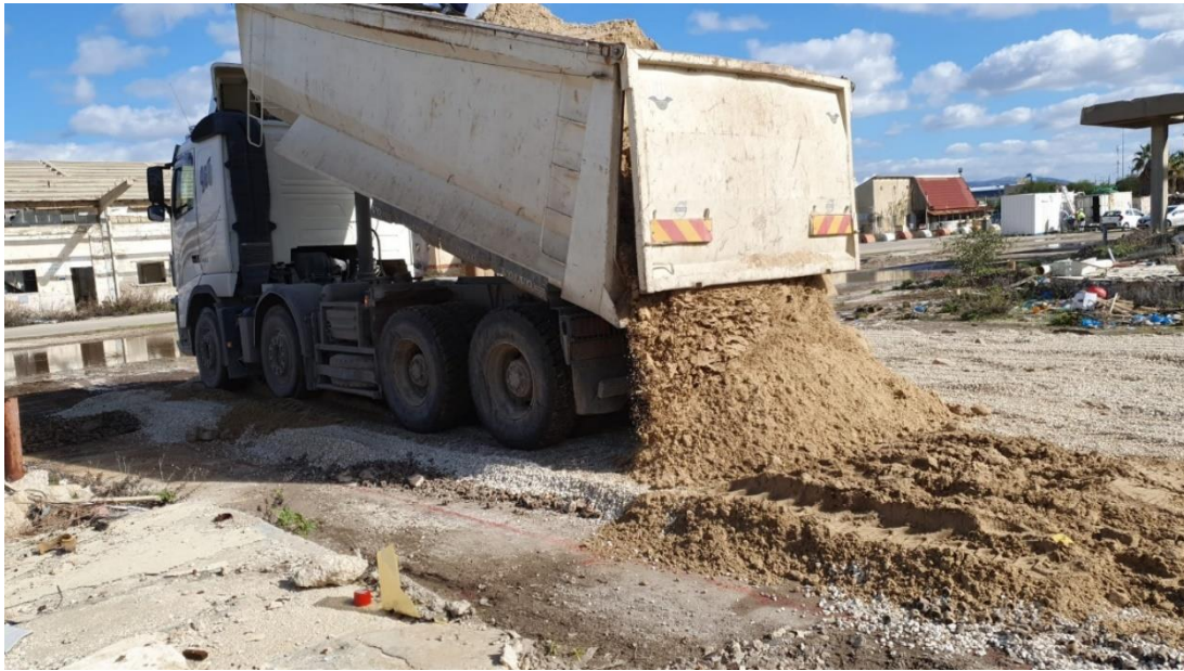
Figure 24. First layer of contaminated soil on the draining bed of the thermal pile
