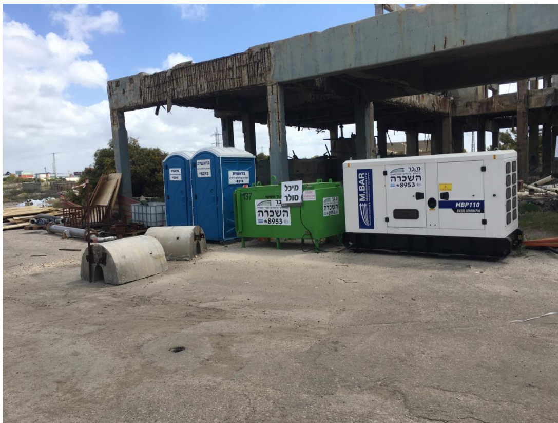
Figure 33. Diesel generator. Green tank: diesel tank, white container: generator
