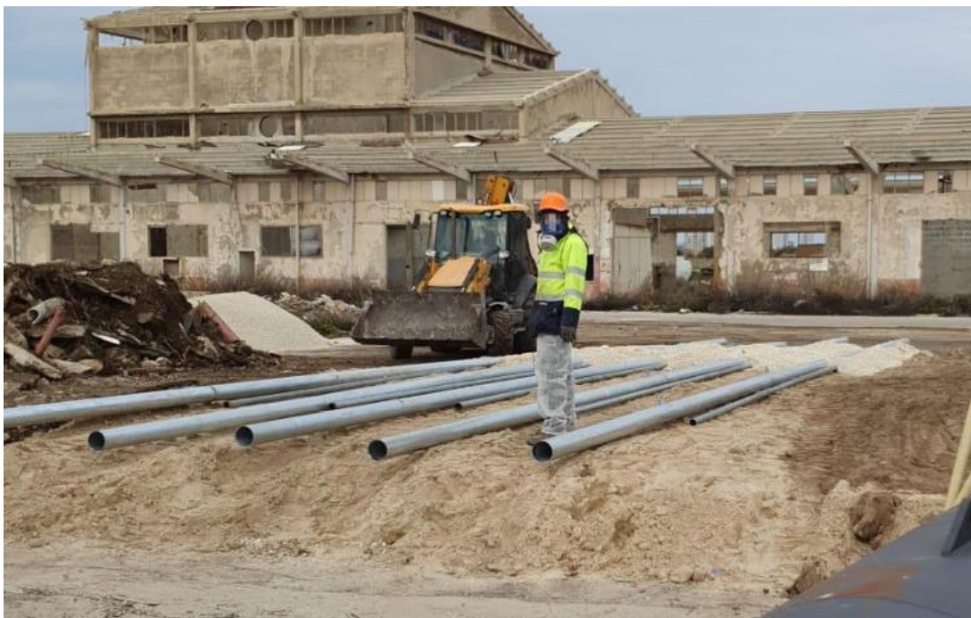
Figure 25. Installation of the first layer of heat exchanger tube
