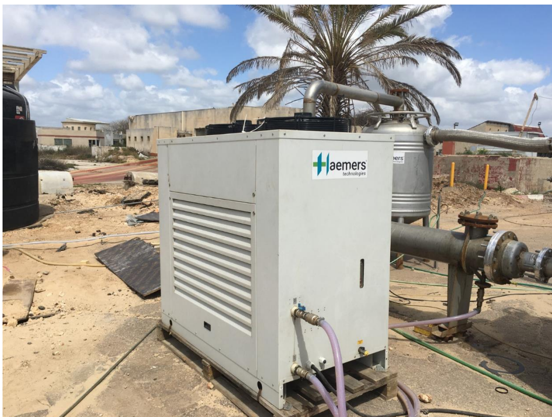
Figure 35. Chiller connected to the second heat exchanger
