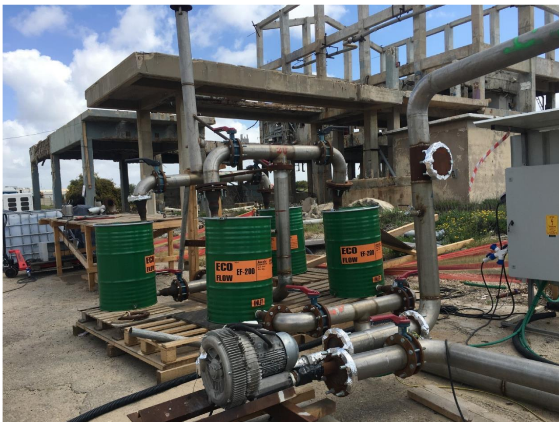
Figure 37. Activated carbon barrels in series to trap the non-condensable VOC and mercury vapors
