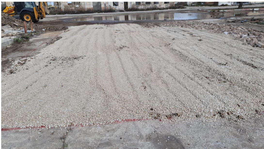
Figure 22. First layer of draining bed
