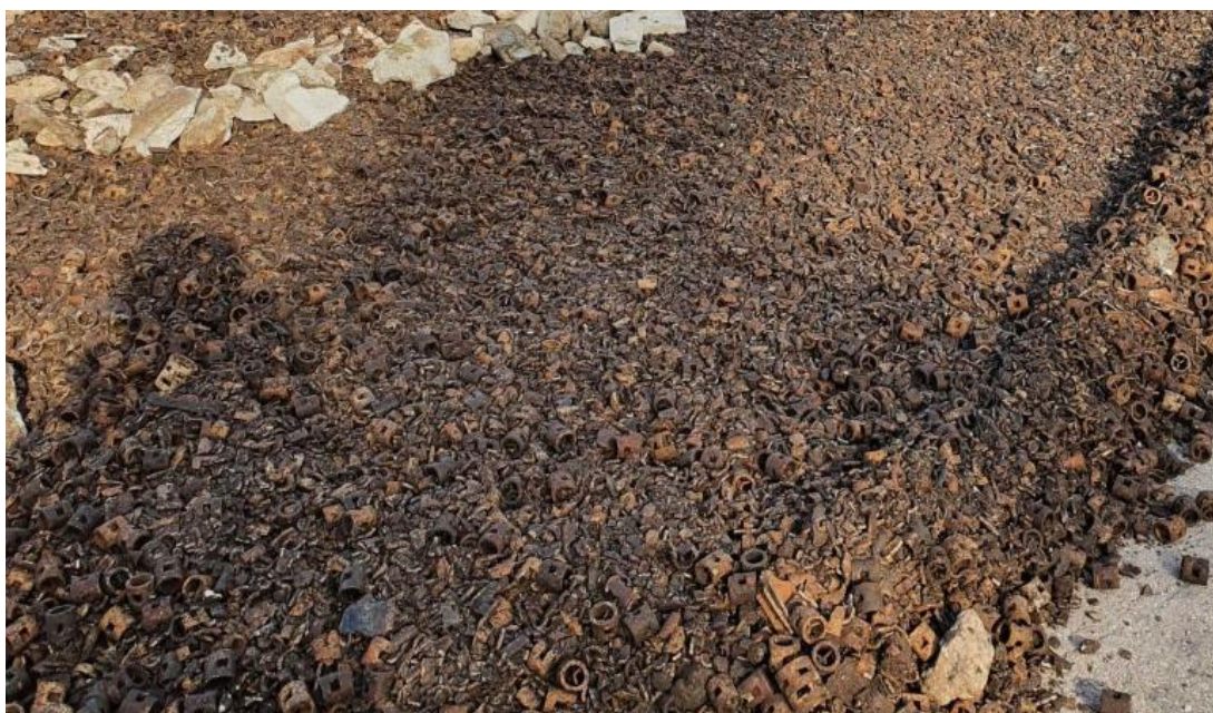
Figure 23. Second layer of of draining bed of thermal pile
