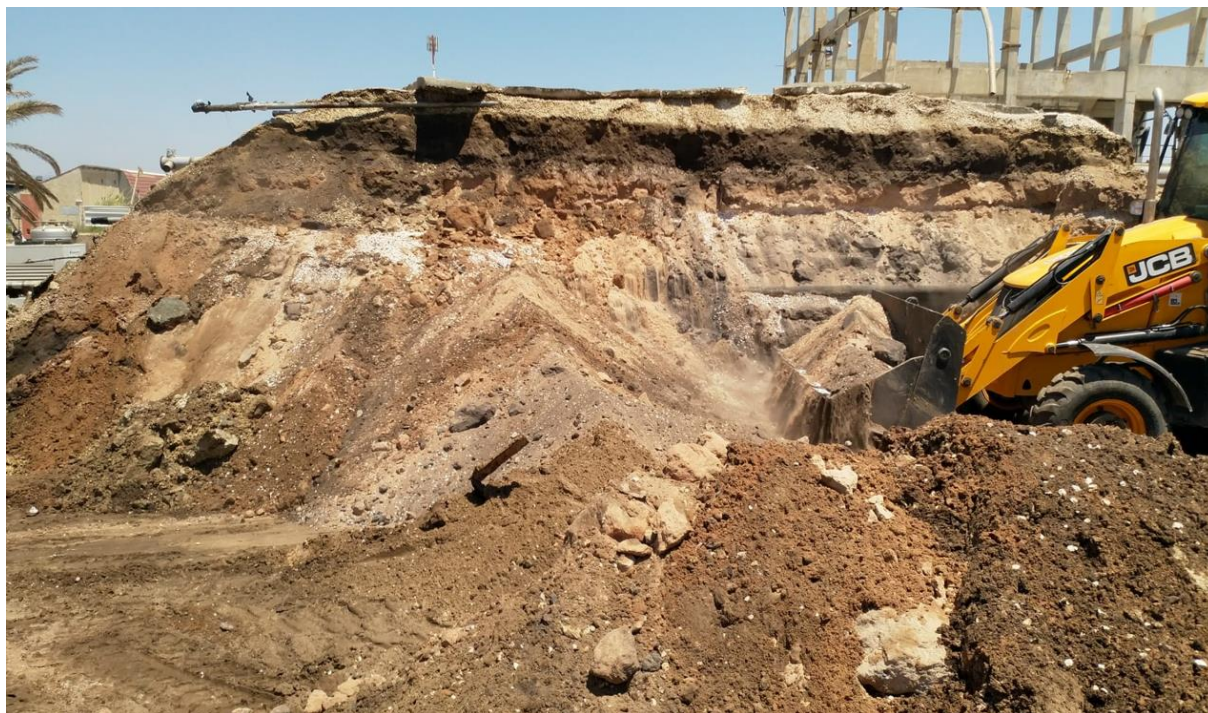
Figure 56. Dismounting of thermal pile
