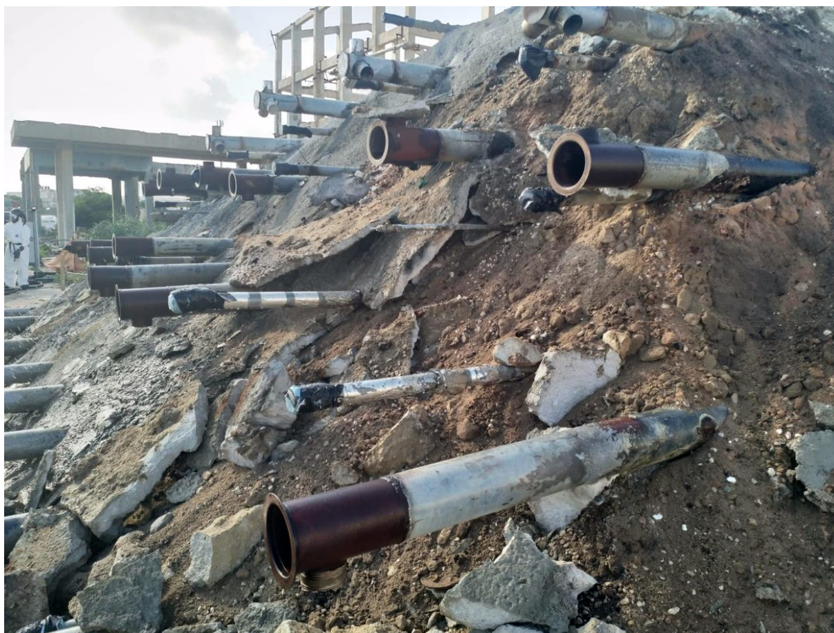
Figure 53. Concrete slab removal on the pile
